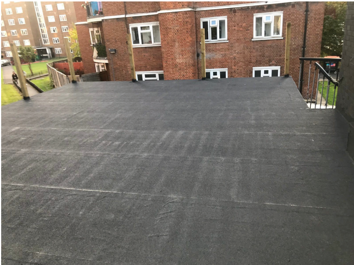
Completed roof, finished with acoustic felt:
